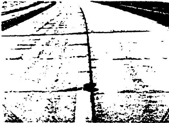
Fig. 3.2.3.7 — Joint separation
